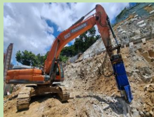
採用組合式隔音墊及 調諧質量阻尼器 Adopting a New Combination of Acoustic Blanket and Tuned Mass Dampers
