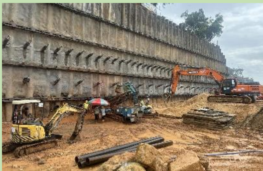
擋土牆打樁工程 Piling Works for the Retaining Wall
